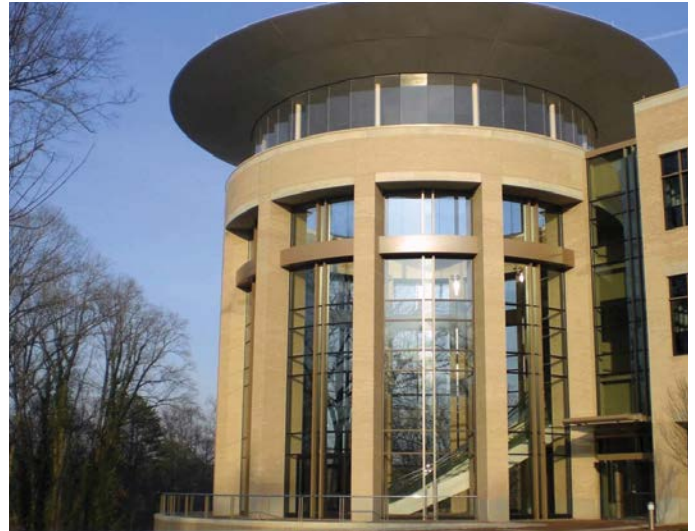
Greenville Hospital System Rotunda Greenville, SC
