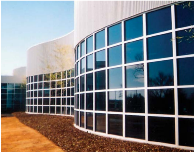
Hyundai Training Center Montgomery, AL
